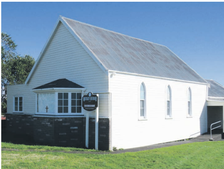
The Rahotu Church and its rusty roof.
